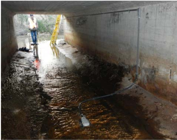
SonTek IQ acoustic Doppler profiler based open channel/ non-full pipe flowmeter being installed in a typical stormwater culvert.
